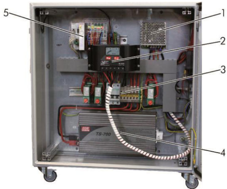
Figure 3-2 Components of the front side of the cabinet
